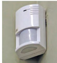
**10 FRESH AIR MONITORING** High carbon dioxide levels in the air (caused by people breathing) make you feel tired and are unhealthy. Carbon dioxide (CO<sub>2</sub>) sensors in classrooms and meeting rooms provide fresh air whenever CO<sub>2</sub> levels get too high. These sensors also save energy by powering down heating and air conditioning when the space is empty.
