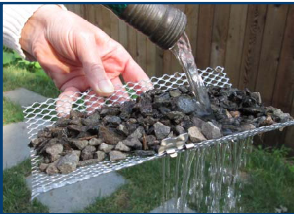
Step 2: Retrieve the gravel from the shopvac, sift and wash it to remove the dirt and debris (left). Or purchase new washed gravel (right). The gravel must be washed whether you are re-using or buying new.
