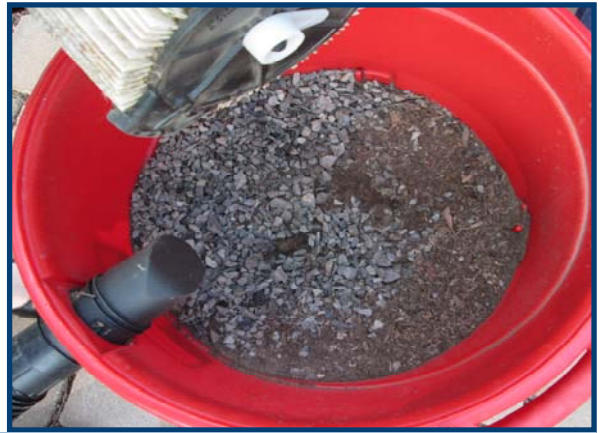
The clogged gravel has been sucked out from between the pavers (left). Gravel and debris inside the shop-vac (right).
