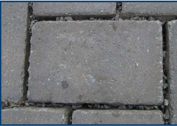
The clogged gravel has been sucked out from between the pavers (left). Gravel and debris inside the shop-vac (right).
