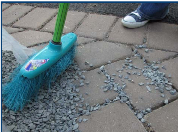
Step 3: Sweep the gravel into the spaces between the pavers. The gravel should be flush with the top of the paver.
